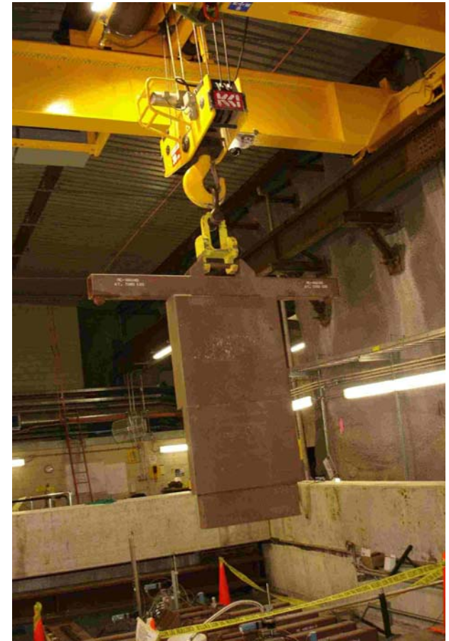
Steel shielding block being moved.
