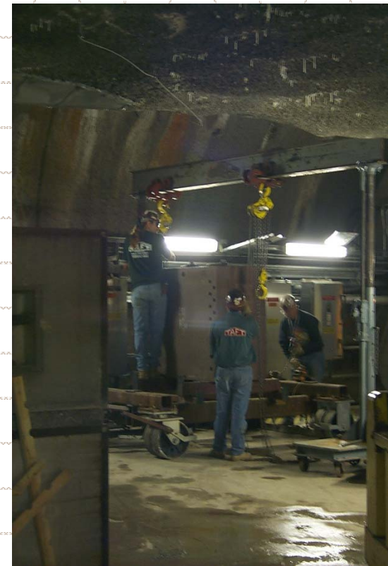
Handling of Shielding Blocks
