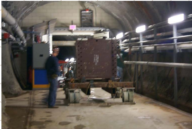
Handling of Shielding Blocks
